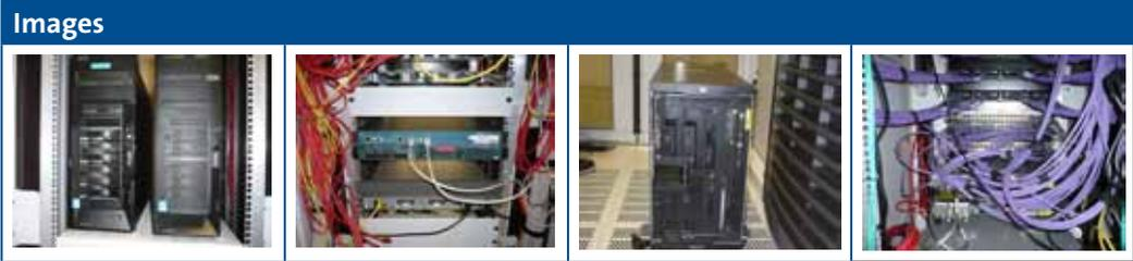
When looking at the installed equipment one already gets a sense of the possible outcome. Although racks, at delivery, are provided completely with blanking panels, brushes and some other measures to seal cabinets, the reality is that over time a lot of those products tend to disappear. The result is a Cold Corridor that has a lot of areas where cold air can bypass or hot air can recirculate.
